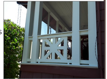
Repainted porch woodwork
